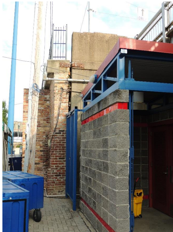
Condition Photo 7: Repaired north abutment backwall separation from the wingwall.
