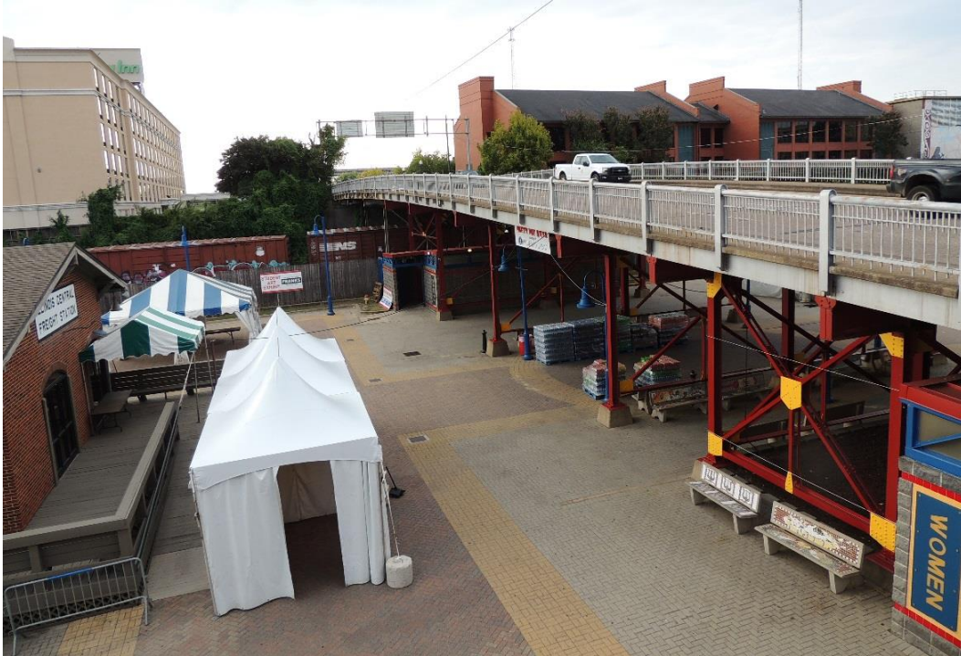
Condition Photo 12: Elevation view looking south of spans 3 through 10.
