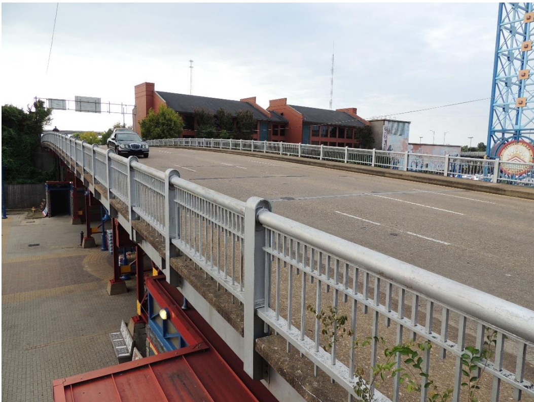
Condition Photo 13: Elevation view of railing looking south.
