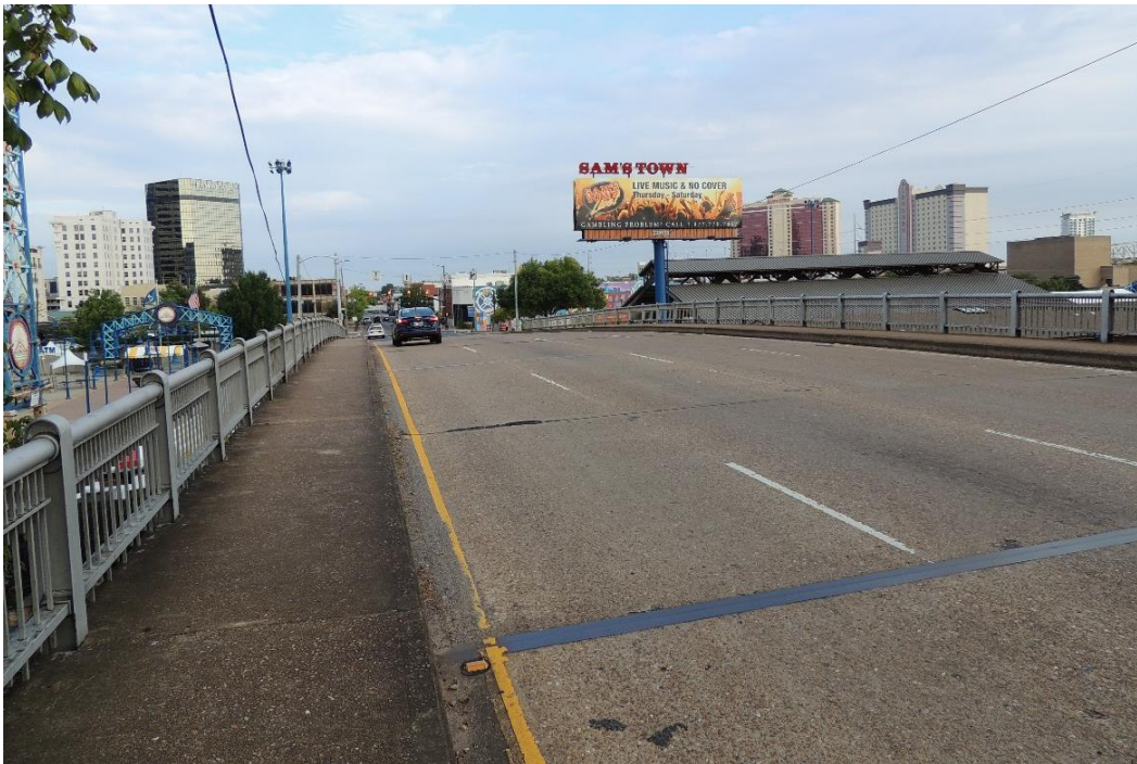
Condition Photo 1: South bridge approach looking north.
