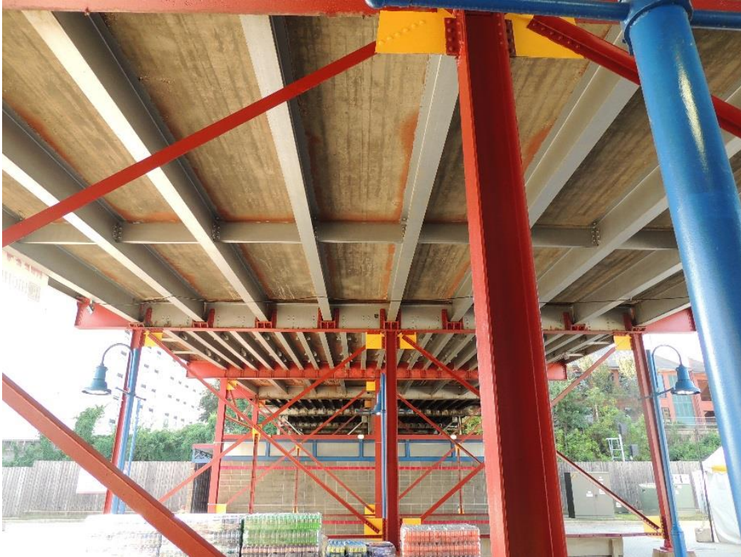
Historic Fabric Photo 2: Steel interior bents and bracing, view to south.
