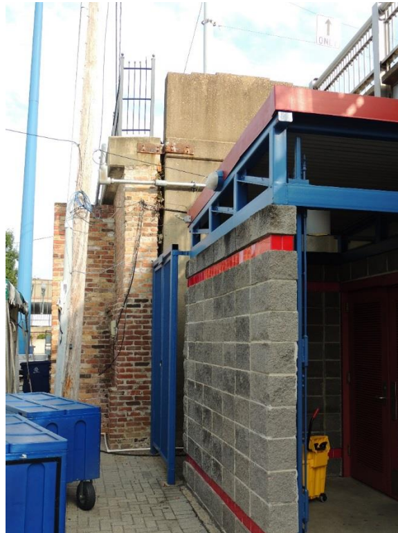
Historic Fabric Photo 1: Reinforced-concrete abutment, partially obscured by a restroom facility, and brick wingwall on north end of bridge.
