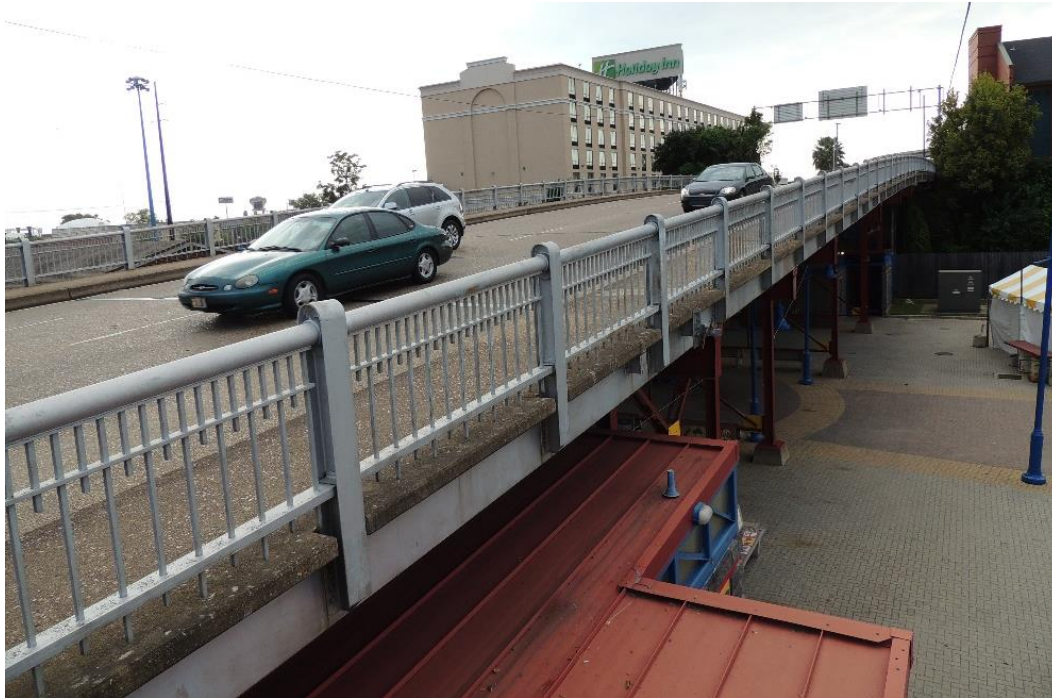
Historic Fabric Photo 4: Original metal vertical picket bridge railings, west elevation.
